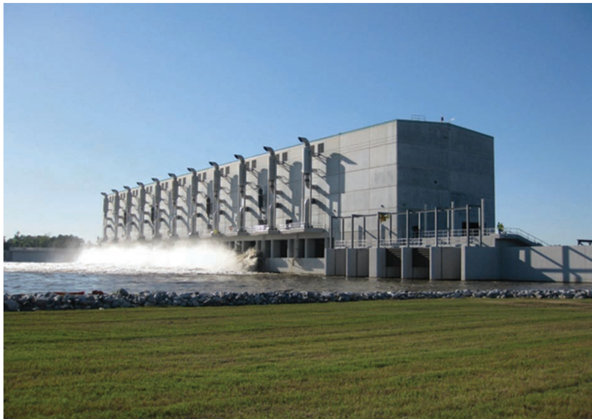
Pompstation van Arcadis in New Orleans
